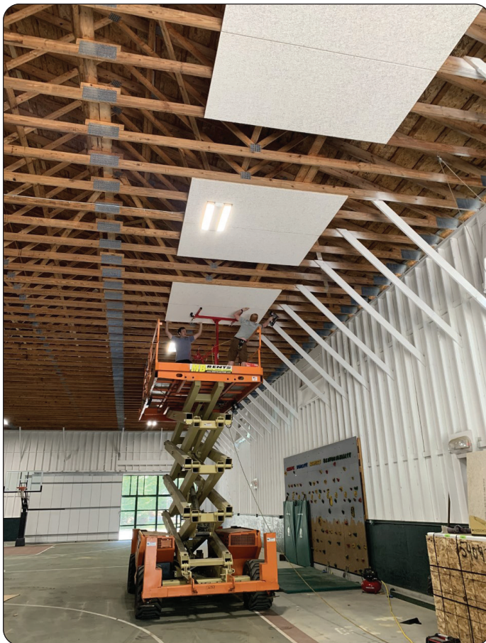
Acoustic panels have made all the difference at the Snell Dome.
