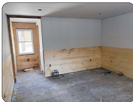
Freshening up the staff bungalows.
