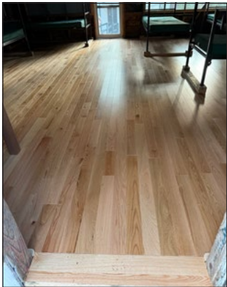
Replacement cabin floors in the Middler and Senior Cabins
